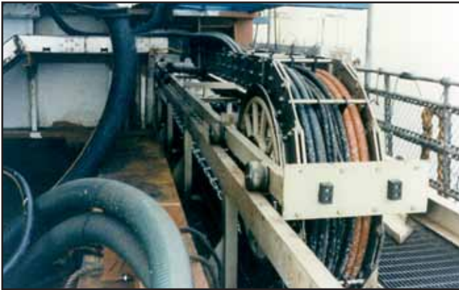
Product: VARITRAK S Operating Mode: Horizontal (long travel, rolling carriage system) Application: Petrochemical Production Equipment 112
