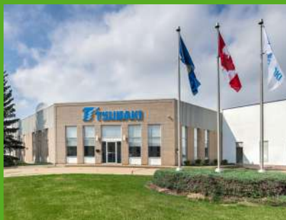
Edmonton Office & Warehouse
