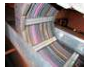
Guide channel installation
