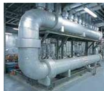
This heat exchange system cools our injection molding equipment with heat from an electrical generator.
