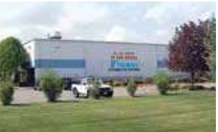
UST Chicopee Plant
