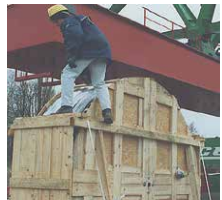
■ Assembly of the fully harnessed cable carrier system
